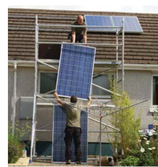
Number 17 - fitting photovoltaics
